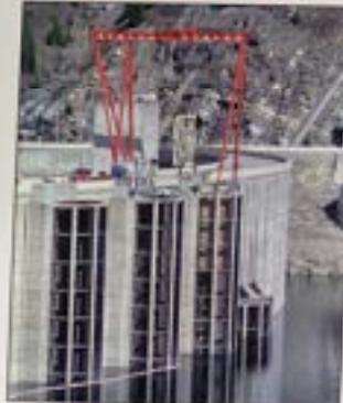
In 1992 Hungry Horse Dam was retrofitted to allow selective withdrawal of water from the reservoir. These gates can be adjusted to draw warmer water from near the surface of the reservoir to release down stream, benefiting native trout.
